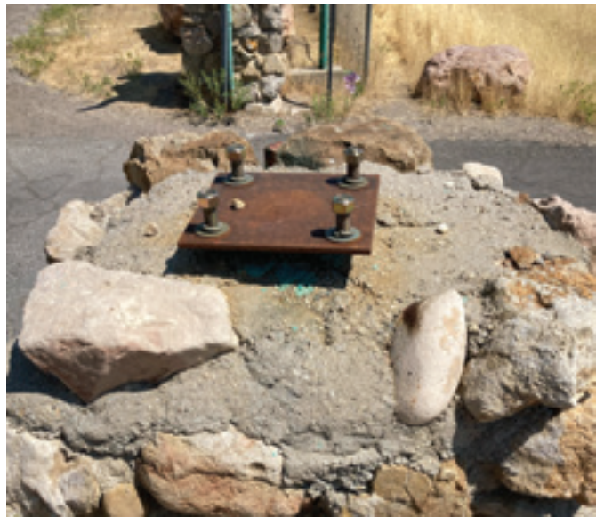
EXISTING STONE PILLAR DETAIL
